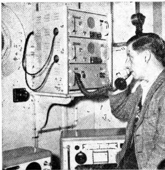
A by-product of the Redifon GR174 a.m. f.m. radio-telephone equipment is that it gives the marine user the opportunity to overcome interference should other vessels nearby be operating on a.m. on the same frequency. The combined a.m./f.m. 20-channel radio-telephone is shown installed in a deep-sea trawler.
